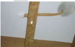
Chrysotile paper on strawboard ceiling panels
