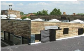
AIB fascia panels with wood effect finish
