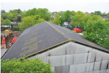
Asbestos cement roof and cladding
