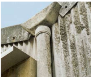
Asbestos cement downpipe
