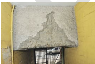
Sprayed coating on building
