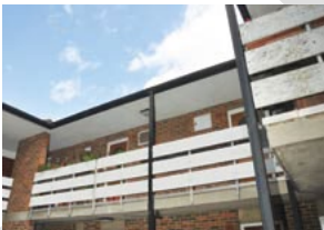
AIB exterior panel on open walkway
