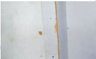
Chrysotile paper on fibreboard boxing
