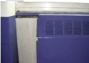
AIB behind school radiator unit
