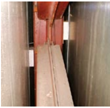
AIB offcuts used as packers around column in CLASP building
