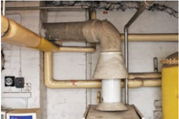
Asbestos cement boiler flue
