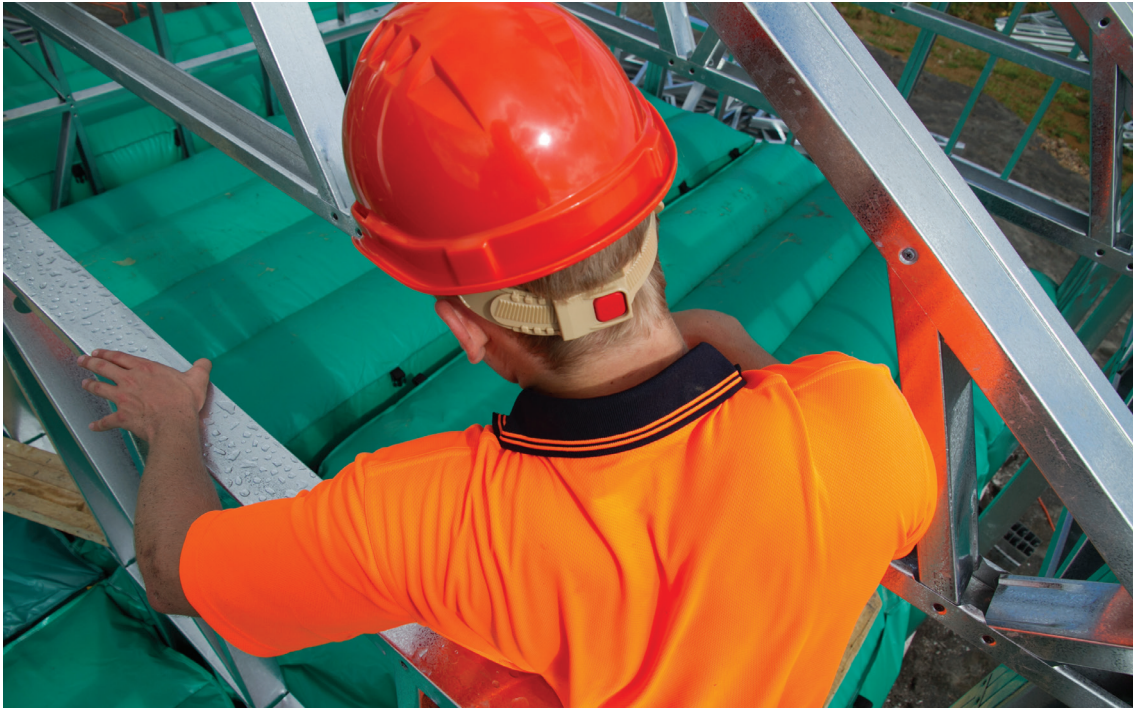
Figure 6: Air bags being used as a fall mitigation measure during roof work (Image courtesy of Airtek Safety Products Ltd).
