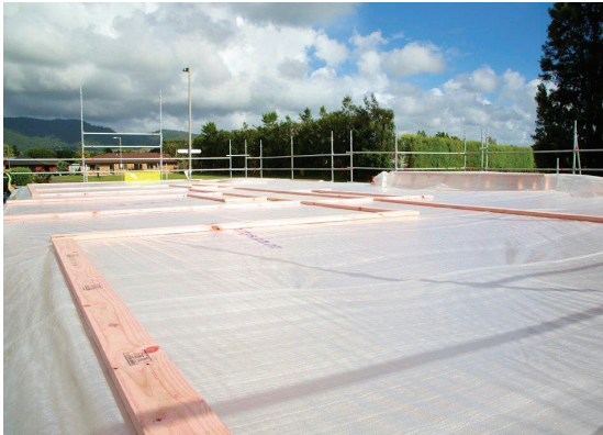
Figure 4: An example of a safety rated product that can span across the top of the framing (image Courtesy of Humpty's Fallbreaker Ltd).
