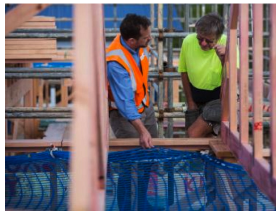
Figure 5: Safety nets installed on a house under construction.
