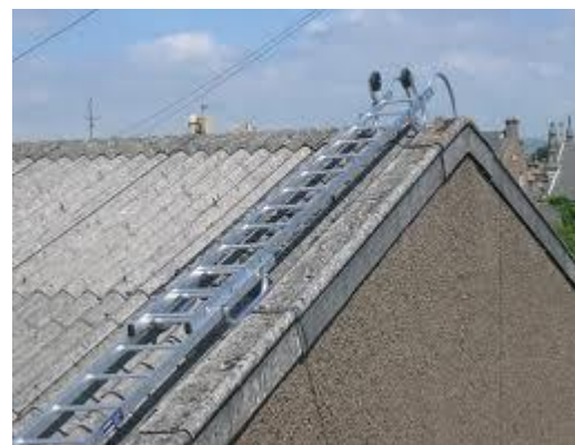
Figure 3: An example of roof ladders on an asbestos roof.
