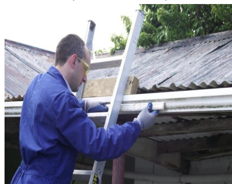
Figure 1: A worker maintains three points of contact while working from a ladder.
