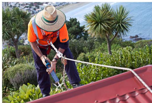
Figure 14: Minor roof repairs can be undertaken using a work positioning system.
