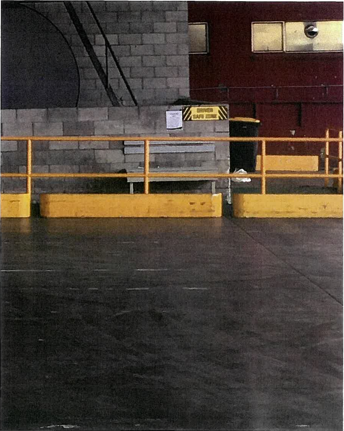
Driver Safe Zone Door 40 – Linehaul Loading on grade
