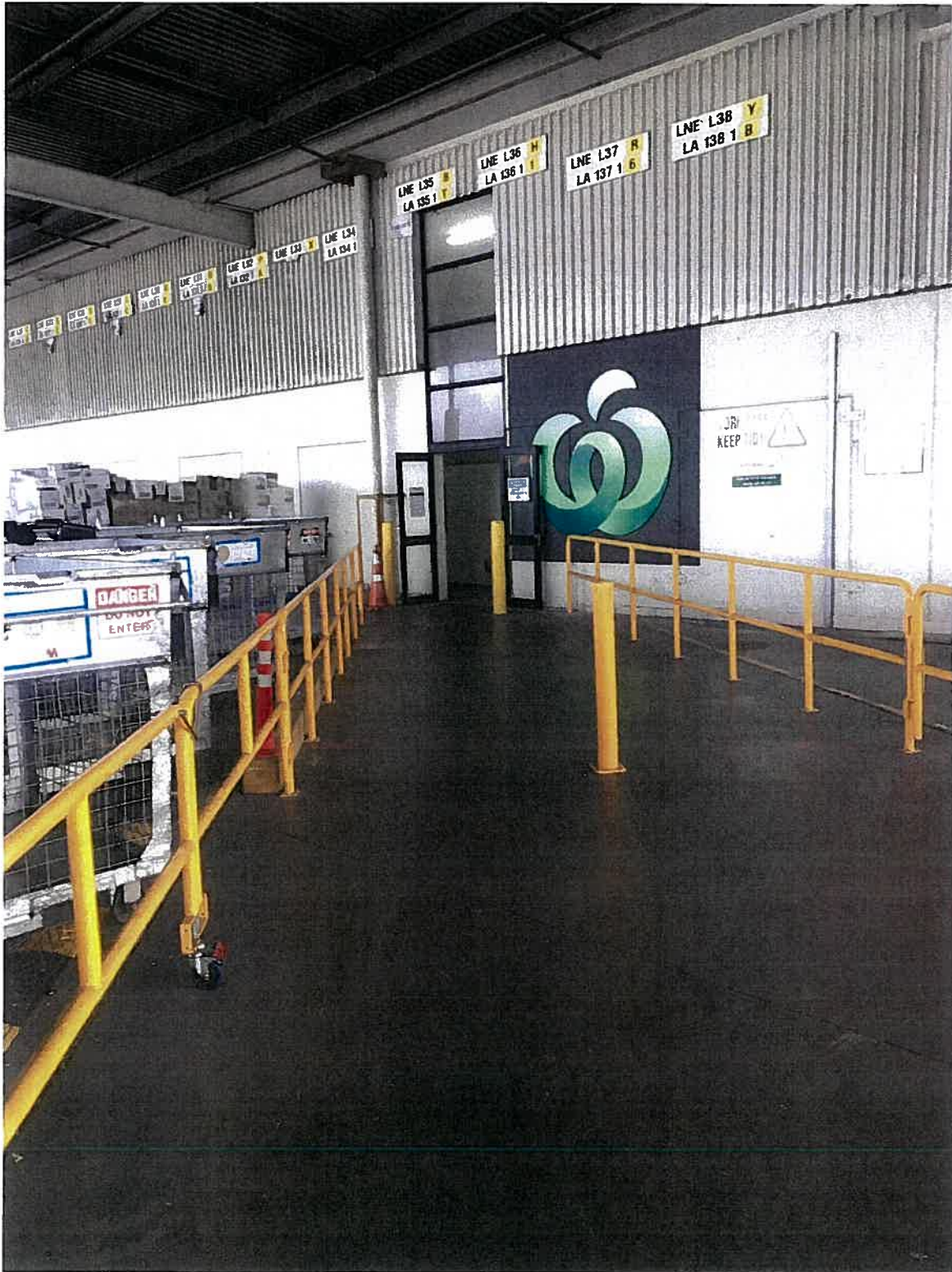
MHE / Vehicle – Pedestrian Separation – This is the main entrance way into the DC for all team members.
