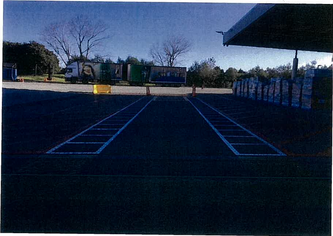
Painted line marking to indicate truck placement as well as person movement and forklift zones around a truck at Doors 39, 40 and 41
