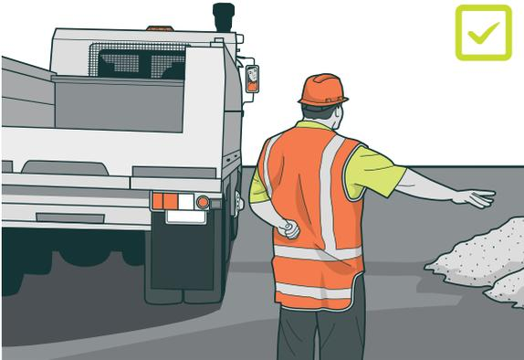
**FIGURE 7:** The correct place for a spotter to stand
