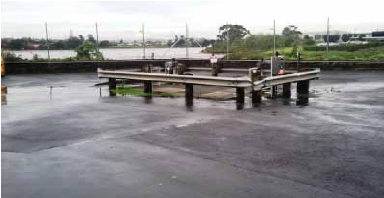
In this example, the entire site is hard paved with a perimeter concrete nib wall. There are individual ramped storage areas within the site where localised spills are trapped. The site's surfaces outside of the storage areas are contoured to this catchment and sump area. The float switch of the pump has lockouts driven from analysers for contamination.
