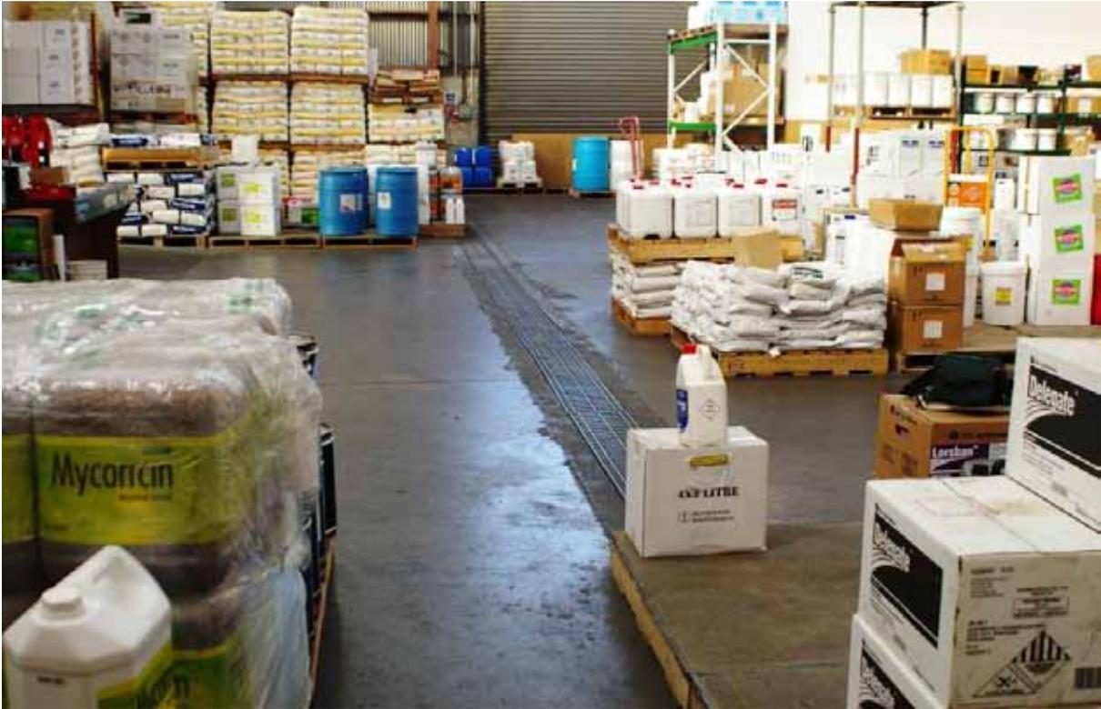
This store has a surrounding nib wall with entrance ramps and contoured floor. The centre drain slopes to an internal sump where it can be pumped out. The store is attached to a retail shop and has electronic keyed entrance.
