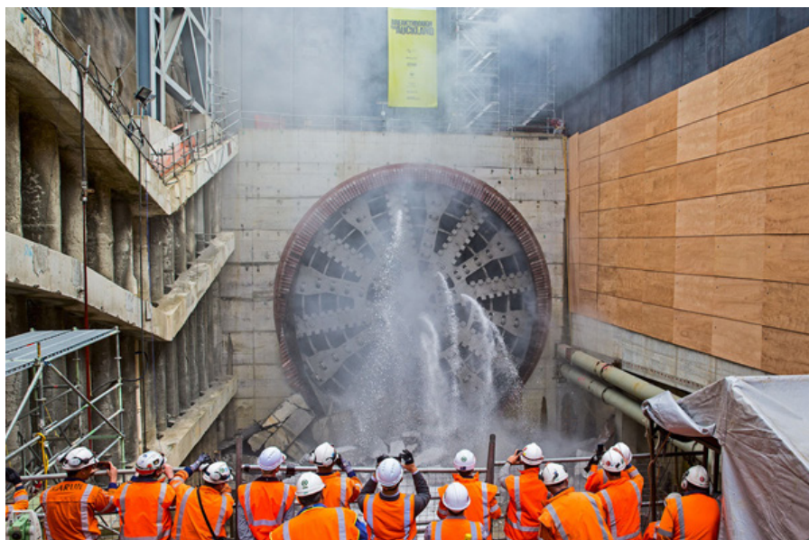
TBM Breakthrough at the Southern Portal
