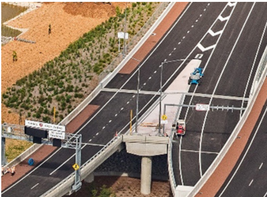
Close-up of infill slab and 'see through'
