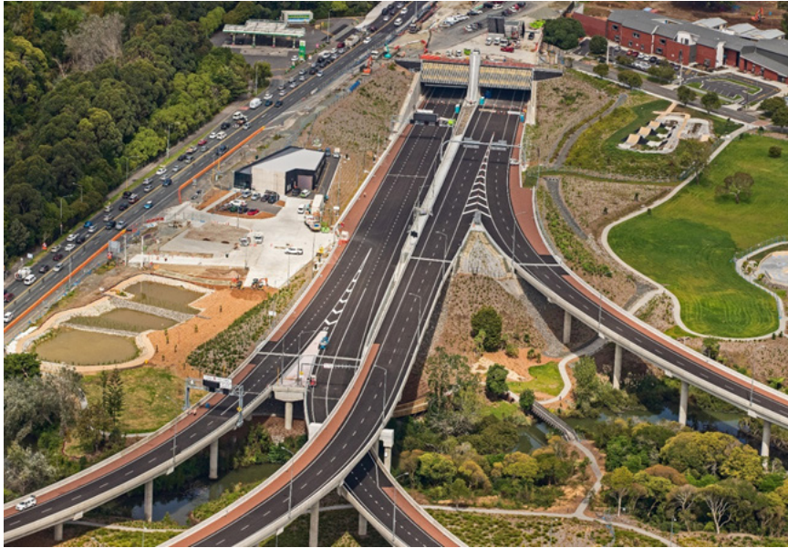
Southbound merge approach into the northern
